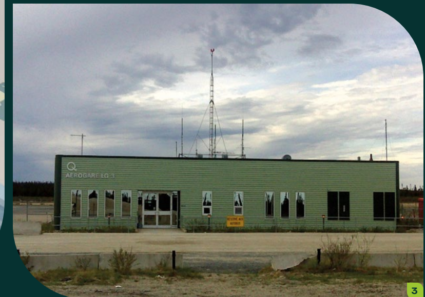
3 Hydro-Quebec's LG3 Airport, James Bay, QC
