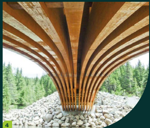
4 Award winning timber arch bridge made of local eastern spruce allowing for a 44% reduction in greenhouse gases (GHG) compared to a conventional structure
